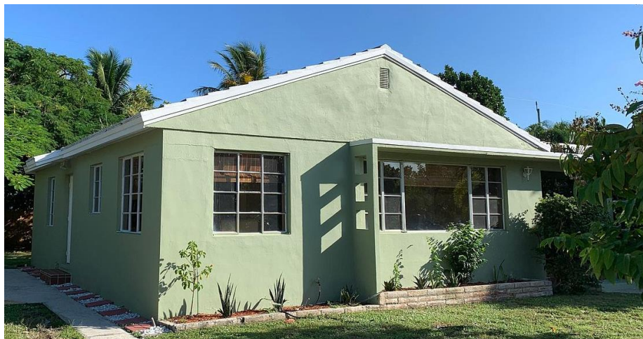
Existing Flat Concrete Tile Roof
